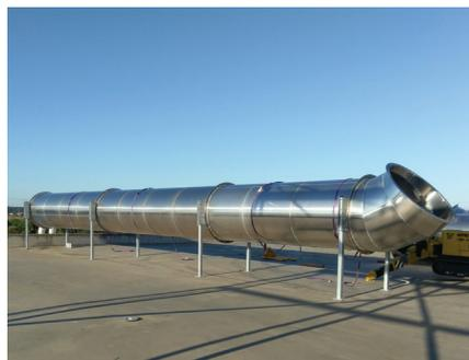
An aluminium air extraction duct being installed on top of the main building
